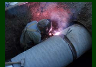
Nick Bezates welding away on the Georgia Pacific-Toledo Project
