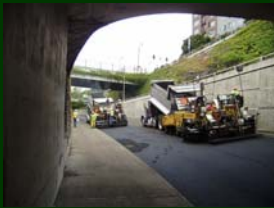
Paving on I-405
