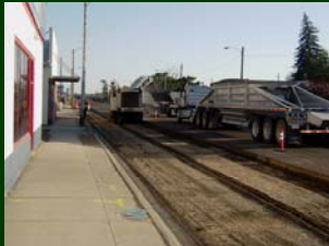
Milling Crews at N. Oregon Street.
