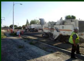
Loren Ziebert and the milling crew hard at work
